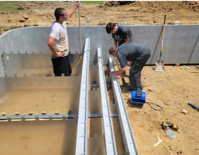
Easily Modified On-Site Tread panels can be cut to custom widths using standard tools
