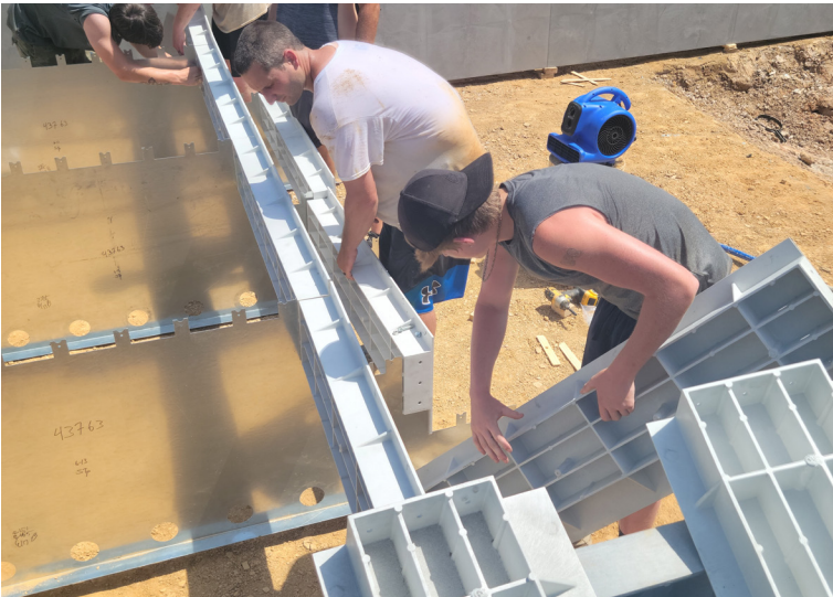
Lightweight and Easily Assembled Tek screws and bolt locations are molded in for fast alignment and secure fit
