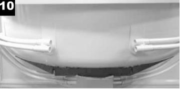
Working on the right side repeat steps 6 through 9. Only the top middle jet bodies remain unconnected.
