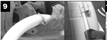
Cut four (4) more pieces of the hose (H02516) to 24" each. Connect the two (2) bottom jet bodies in the same way as the previous two hoses, following the same procedure.
