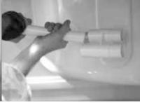
Starting from the left side, connect the air coupling of the top jet to the air coupling to the bottom jet using one of the 52" hoses. Apply PVC cement to each outer end of the hose and the inside of the air coupling just before inserting the hose. **NOTE:** Ensure no glue gets inside of the interior of the jet housing.
