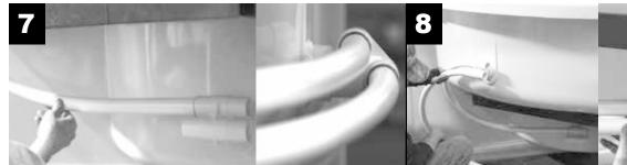
**NOTE:** Make sure to install the line without ANY sag in it. Any sag will cause the jet to malfunction.
